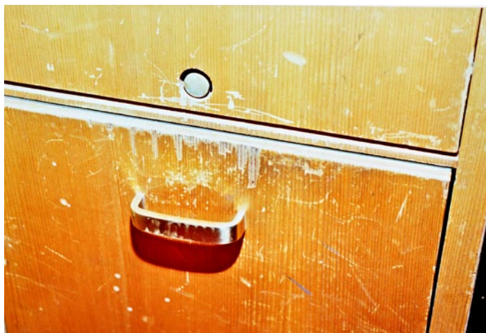
Figure 4. Gordon House filing cabinet showing worn area where finish sample was taken.
