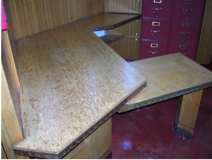
Figure 3. Price Tower secretary's office, 19th floor, before treatment.
