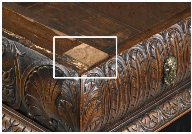
Figure 8. This small block on the interior of the cabinet contained its entire sapwood sequence, allowing the felling date for the tree to be firmly established.
