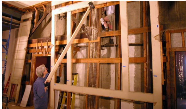
Figure 6. Frame on wall D being lowered to the floor.
