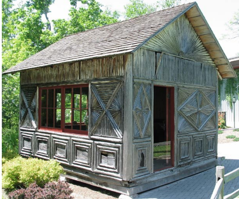
Figure 3. Sunset Cottage, showing pole mosaic with spruce bark inset panels, present condition.
