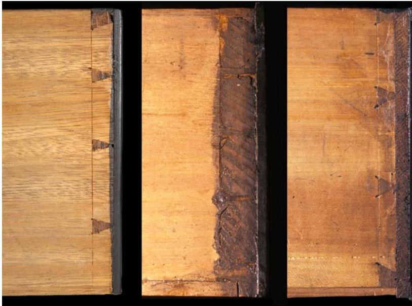
Figure 9. Comparison of drawer construction. Rebuilt drawer (left); an original dovetailed drawer from an ebony cabinet in a private collection (center); an original dovetailed drawer with applied front panel from the ebony cabinet in the Victoria and Albert Museum (right).
