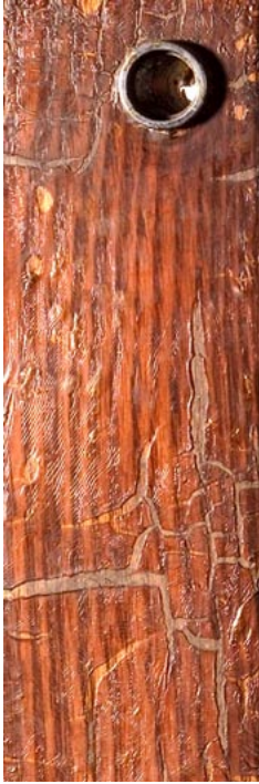
Figure 4. Degraded varnish on the exterior coachwork.
