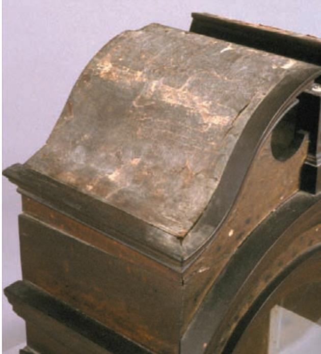
Figure 8. Clock hood showing the paper dust cover.
