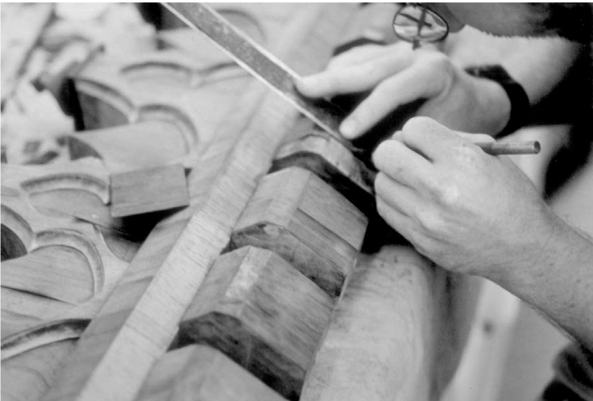
Replacing missing veneers with Brazilian rosewood.
