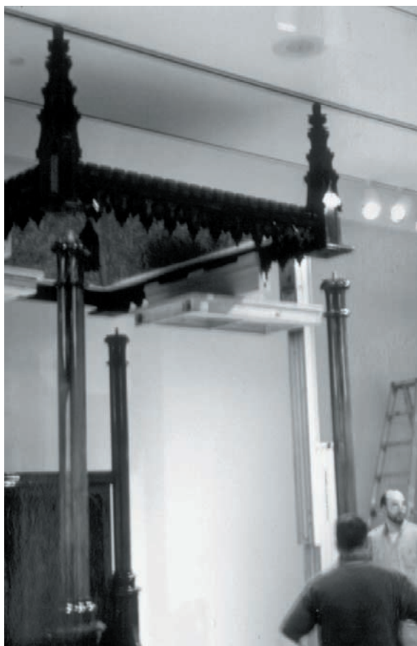
Custom cradles attached to lifts hold canopy in position while bed is assembled underneath.
