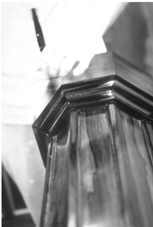
Handbrushing twelve coats ultralight dewaxed shellac.
