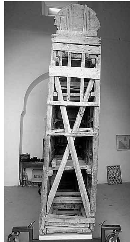
Figure 5: The pronounced list of the minbar. Note existing braces and interior structure.
