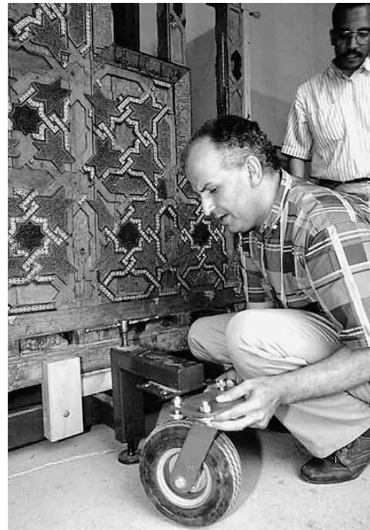
Figure 8: Wheels being inserted into the raised frame. Once attached, the frame could be lowered onto the wheels, and the whole minbar moved about.
