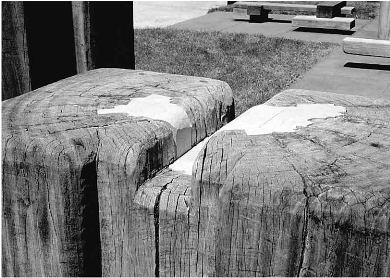
Figure 8: A completed fill showing the Trex insert before its surface color has oxidized.
