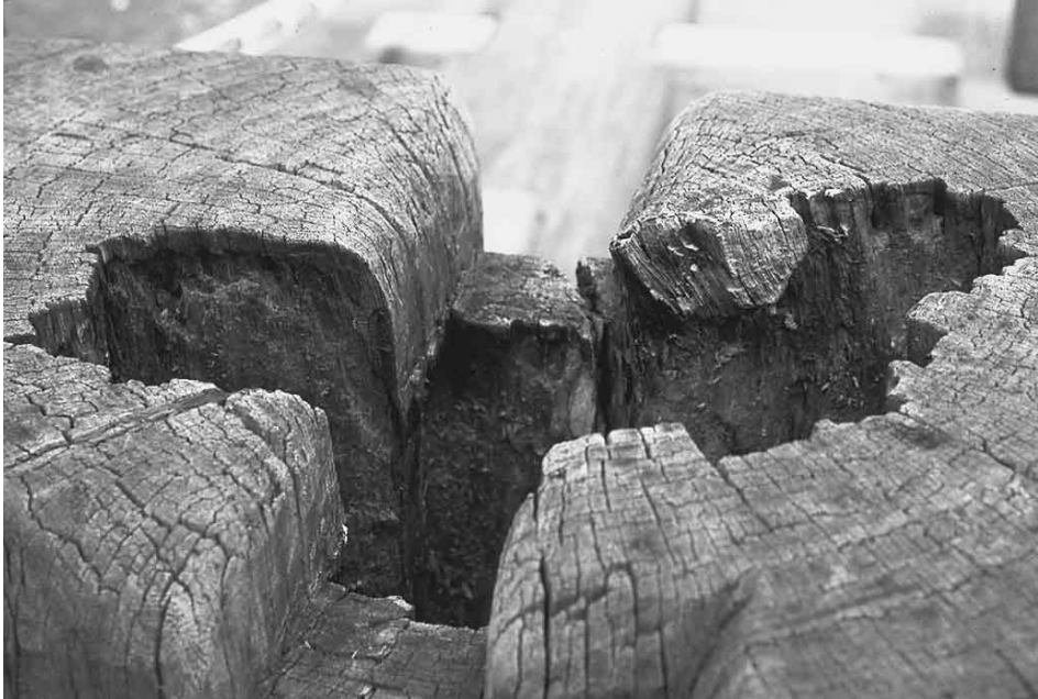
Figure 3: Area of decay in the top of one large center block.
