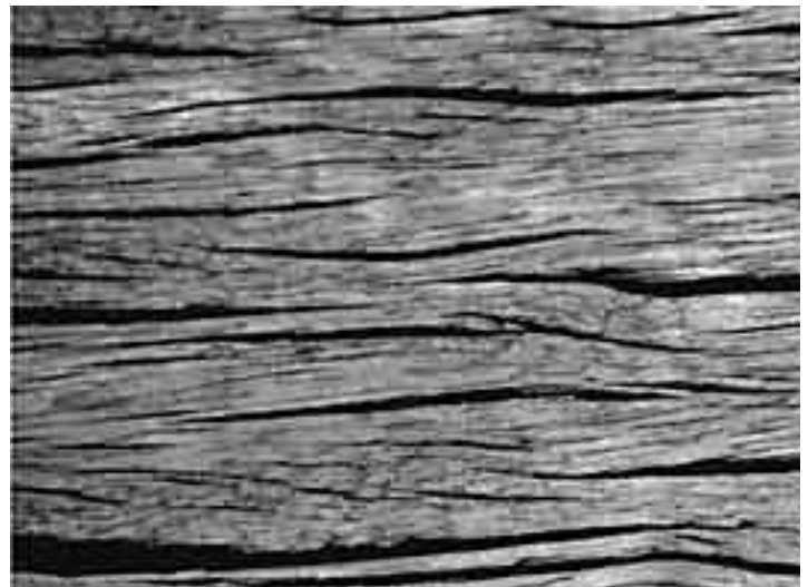
Figure 9: A small Trex fill after its surface has oxidized.
