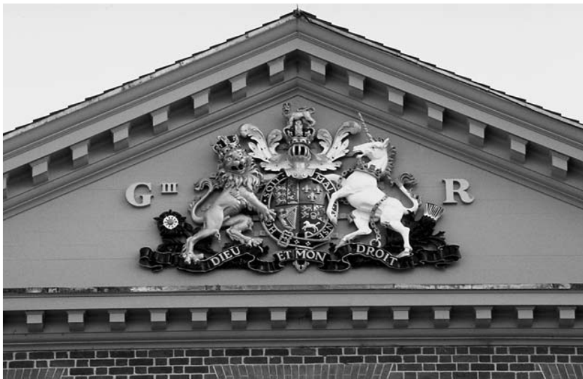
Figure 5. Glass reinforced polyester reproduction.
